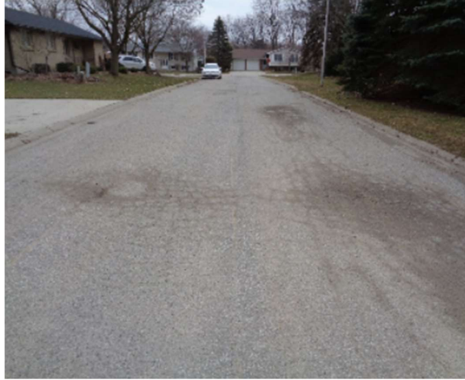
Roadway in Poor condition – serious deterioration, function is inadequate
