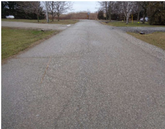
Roadway in Fair condition – deterioration evident, function is affected
