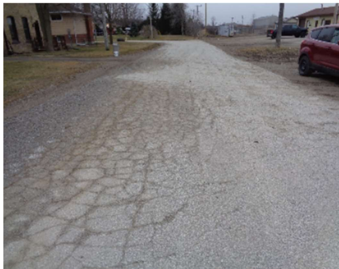
Roadway in Very Poor condition – no longer functional, general or complete failure
