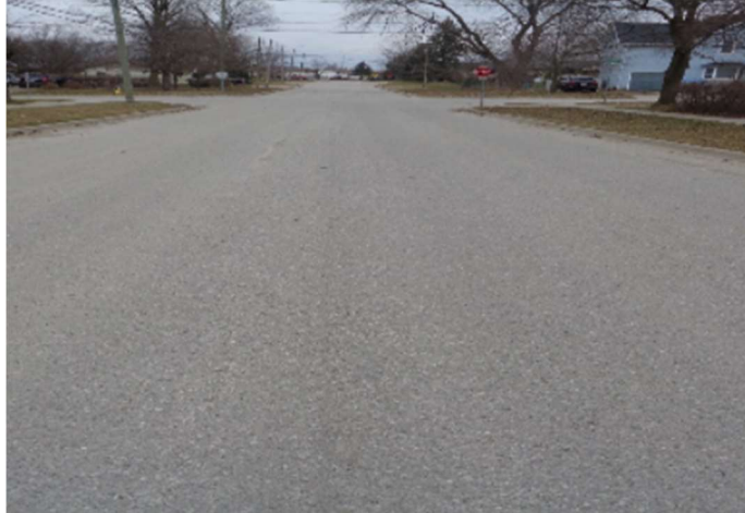
Roadway in Very Good condition – no noticeable defects
